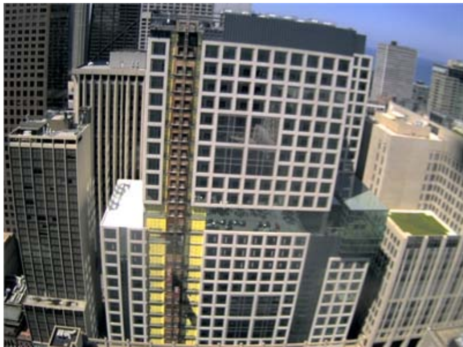
Construction Progress as of July 2010
