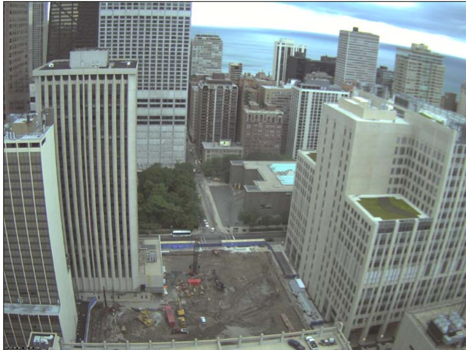
Construction Progress as of April 2008
