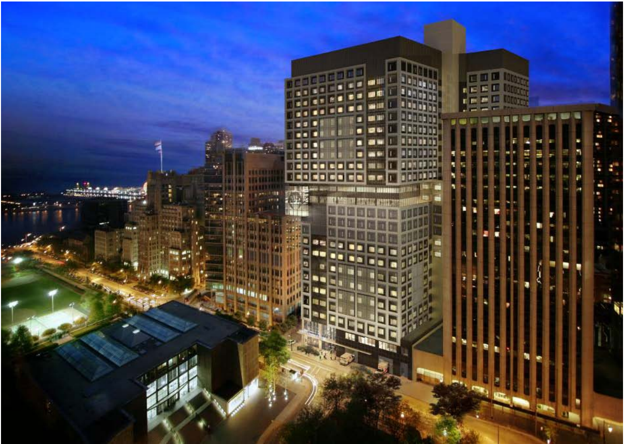
View from Chicago Avenue
